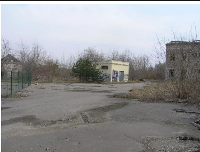
Transformatoru ēka kad.Nr.13000103515002
