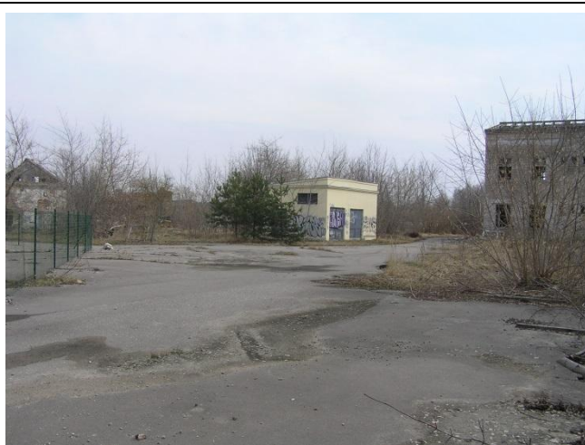
Transformatoru ēka kad.Nr.13000103515002
